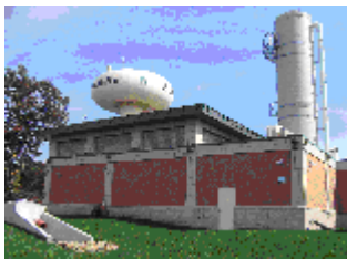
Blaine WTP No. 1
