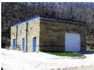
Red Wing Booster Station
