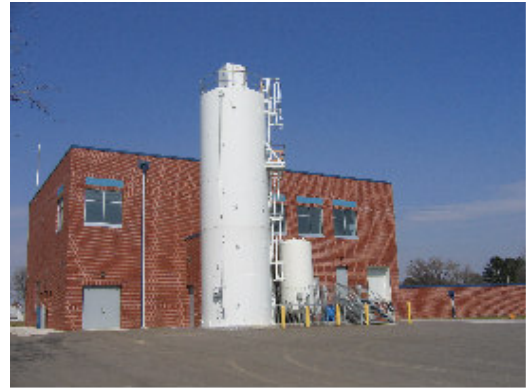
Lime Silo and CO 2 Storage
