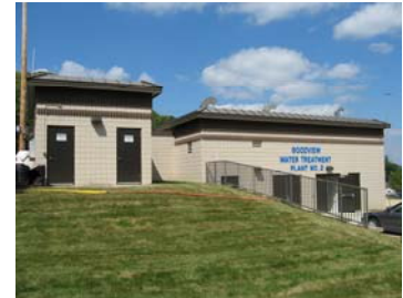
Goodview Water Treatment Plant No. 2
