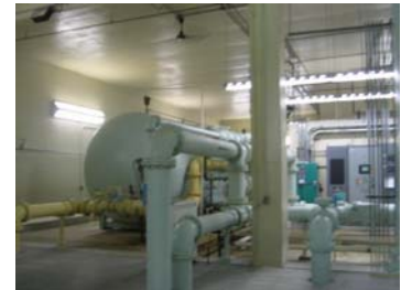
St. Louis Park Water Treatment Plant No. 1
